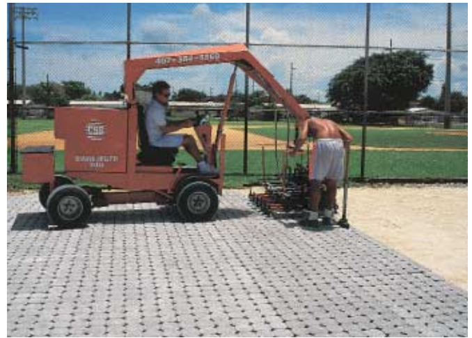
Mechanical installation of UNI Eco-Stone® speeds construction
