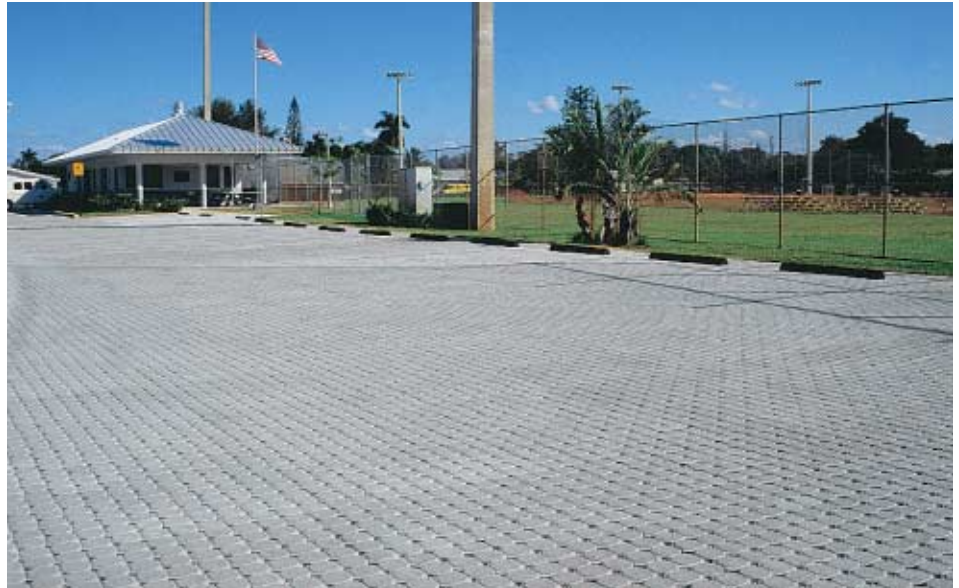
Mickel Field utilizes over 30,000 square feet of permeable UNI Eco-Stone® concrete pavers
