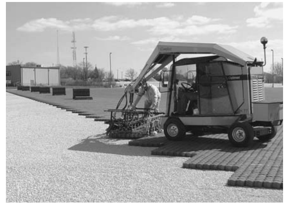
Mechanical Installation of Ecoloc® Permeable Pavers
