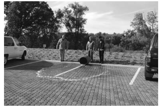
Testing infiltration at the Rainwater Runoff Model
